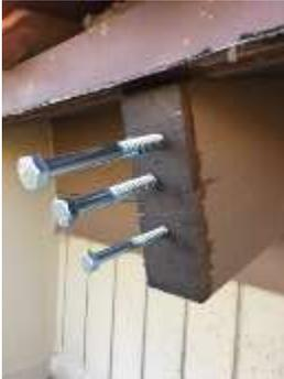
Make a form for pouring new beam ends. This part takes some time to make but is reusable over and over (in my case 17 beam ends)
