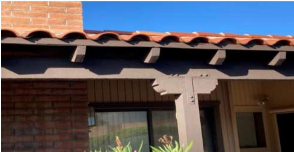
C. If the deterioration has made repair of the existing rafter ends impossible, but you want to preserve the rafter end design, a more dramatic repair is possible. Ed Seale has provided the following pictures and description of the approach he used to maintain the original design.
