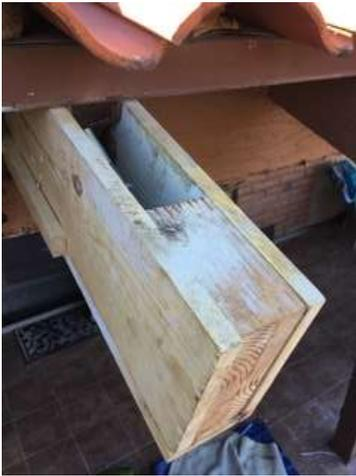
I made a groove between wood beam and new beam end which is filled with silicon caulk to further seal the joint.
