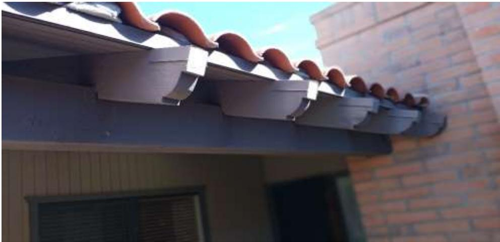
B. If the deterioration has made repair impossible, the Board has approved cutting off the ends of the rafter overhangs. The picture below shows how such rafters should be cut.
