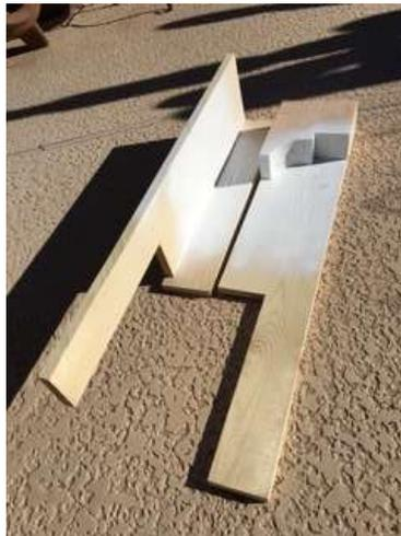
Attach mold to cut off beam end. Pour in mortar mix which flows around lag bolts. When it sets up it locks new beam end in place.
